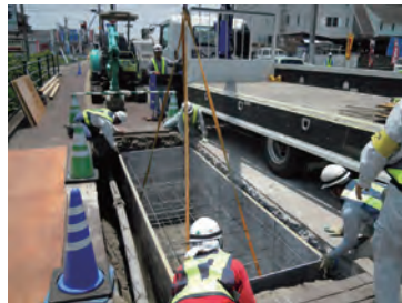
②型枠設置
